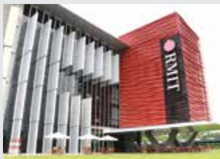
RMIT Vietnam's Academic Building 2 – designed by Pentago Spowers International – reflects the design ethos of RMIT's other landmark buildings in Melbourne.
